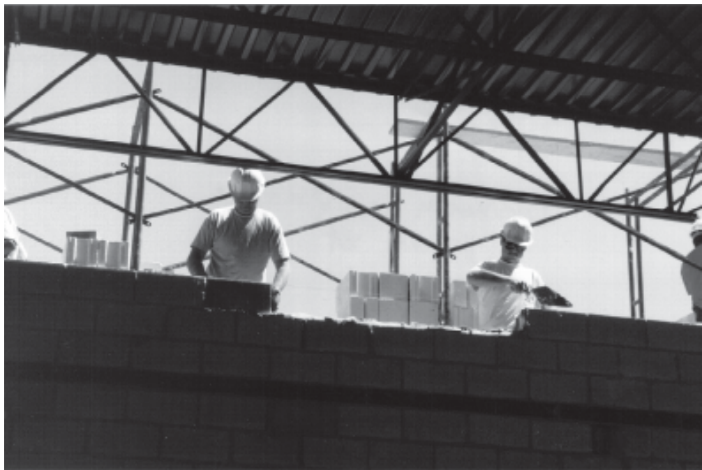
Placement of Concrete Masonry Units
