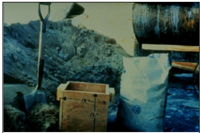
Figure 1—Measuring Mortar Sand Volume
