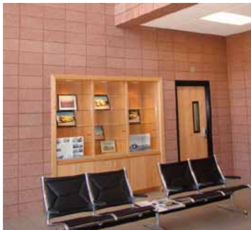
Ground face units with complementary mortar
